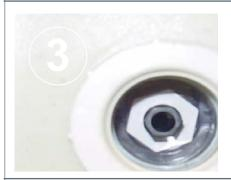
Remove the jet nozzle and nut using a 7/8" deepwell socket and extension.
